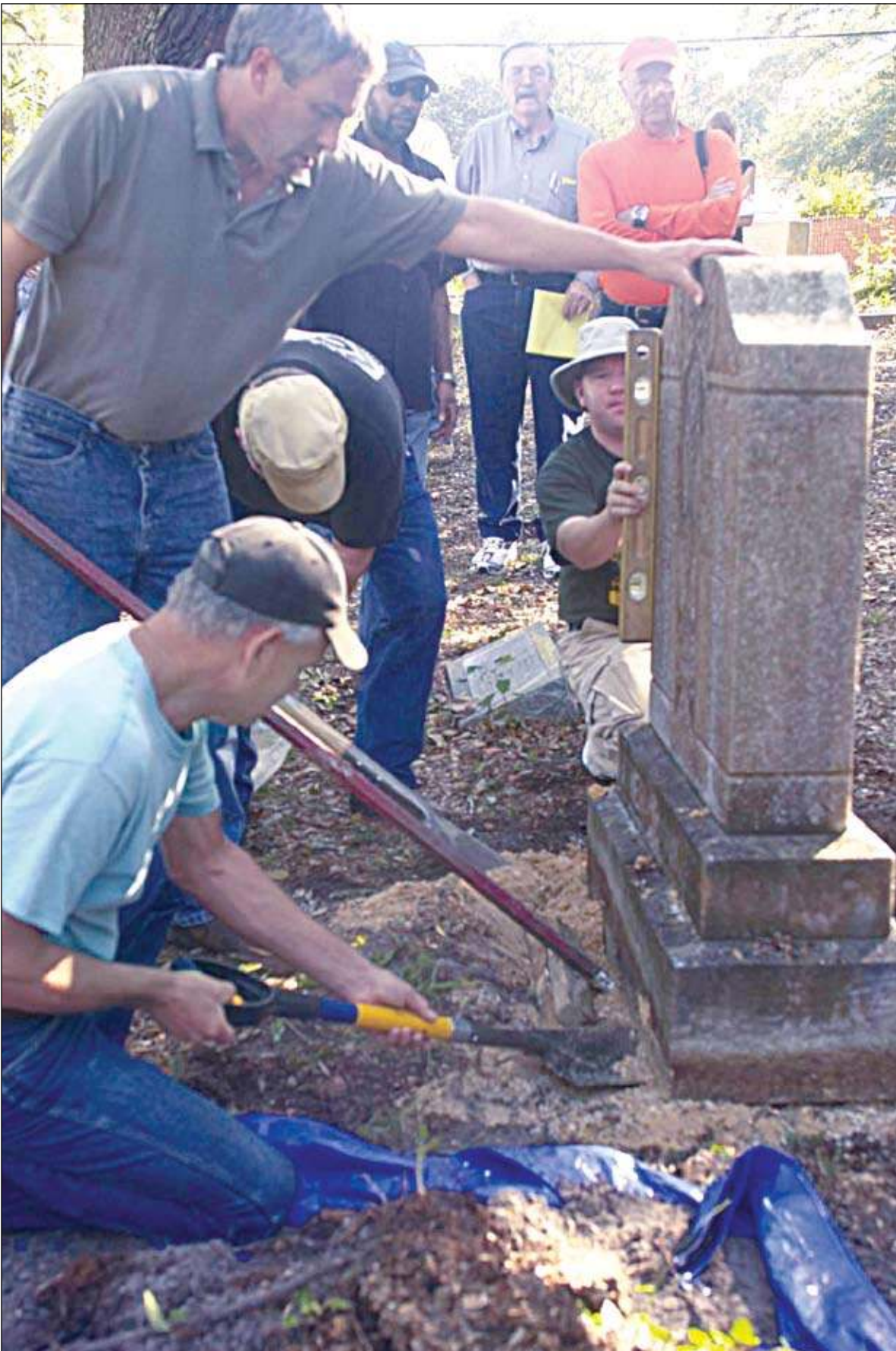
Southport Historical Society member Marvin Johnson pushes loose gravel under a once-skewed grave marker while workshop leader Jonathan Appell uses a pry bar to lift the aging stone.
